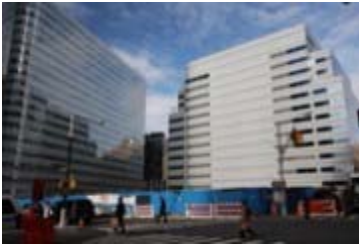
Fiterman Hall site excavated to foundation, December 2009
